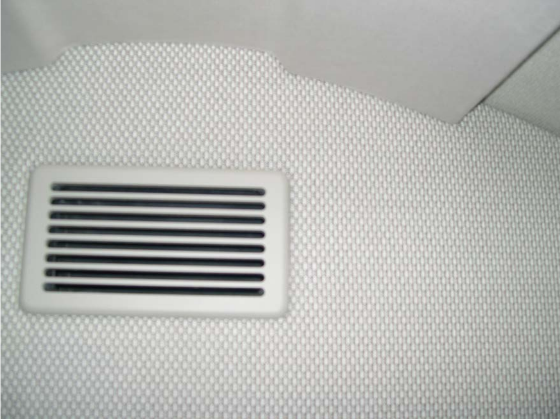
Flood Cooling Door, aft pressure bulkhead
